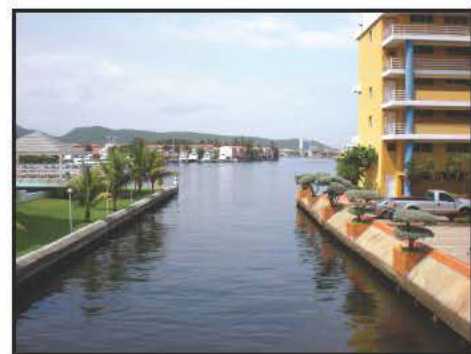
One end of the Horseshoe Canal system. McCiarcia rests just behind the yellow building on the right.
